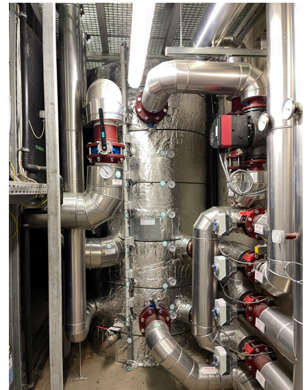
Zortström Multi-PG-H 5-stufig, Durchmesser 1.200 mm, Inhalt 2.940 Liter
