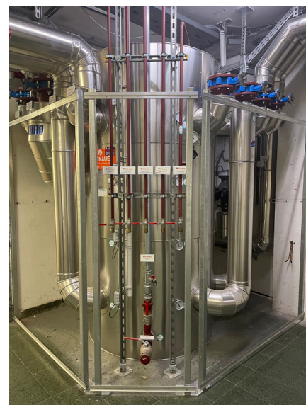
Zortström Multi-PG-H 3-stufig, Durchmesser 1.000 mm, Inhalt 1.690 Liter
